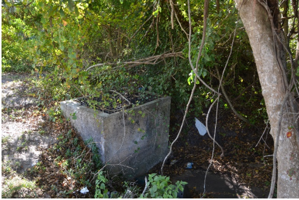
Photo 7: Overflow structure at east end of drainage swale. Only functions at flood stage
