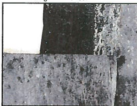
View of Overlap Seam of Dual Pro and Tile Pro
